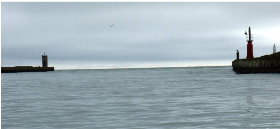
Figure 3-11 The breakwaters and training walls ensure a wide-open mouth (Source: A. Theron).
