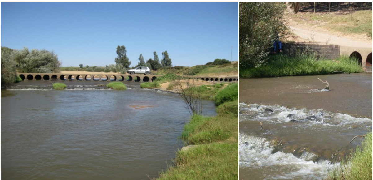
Addendum Figure 9 Klipbank / Doornboom looking upstream towards crossing
