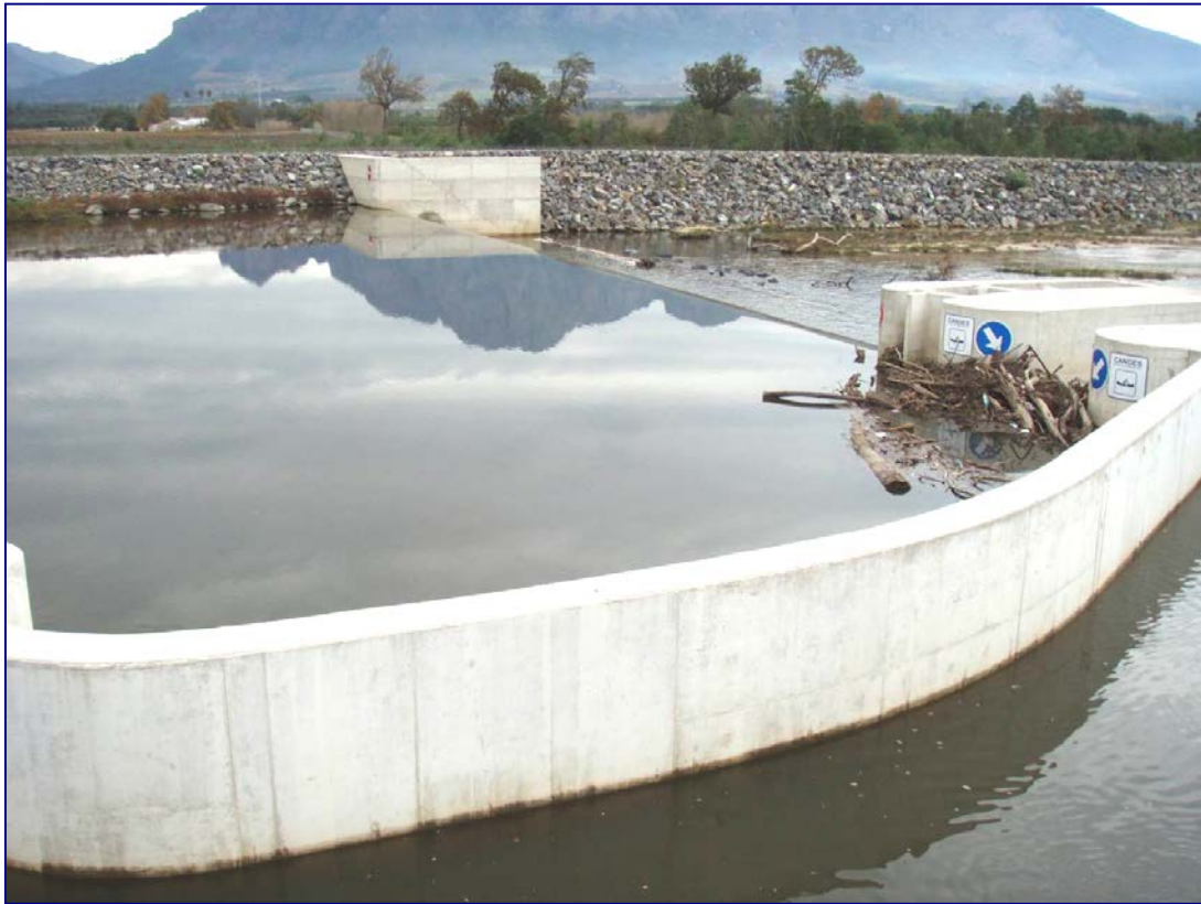
Figure 3-15 Skuifraam Supplement scheme downstream of the Berg River Dam. Note problems with fish ladder and canoe access (Source: A. Theron).
